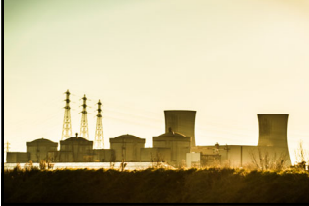
Nuclear Power Plant - x1klima (CC BY-ND 2.0)
